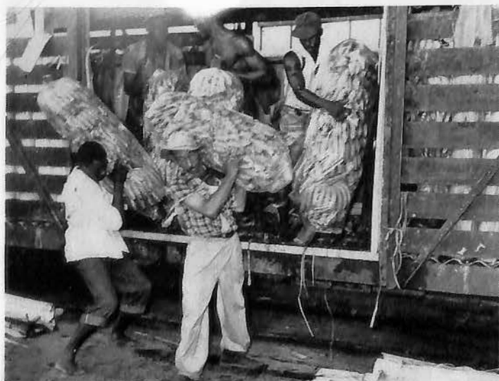
5. UNLOADING cars at shipping docks (this is in Nicaragua). Two interesting points to note are (1) the ends of stems are used as a ski to slide bunches out, decreasing handling; (2) inside of cars is lined with plant slices to cushion the fruit during transport. Clearly, bananas are sensitive fruit.
