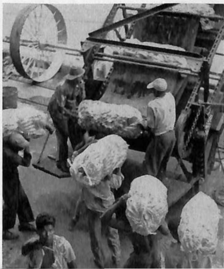
7. BANANAS are being loaded into pockets of gantry conveyor (below), each bunch is counted and graded for size of hands (each bunch on stem is a "hand," individual bananas are "fingers").
